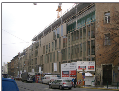
West view of the construction site - 2009
