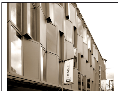
Detail of the façade - 2009
