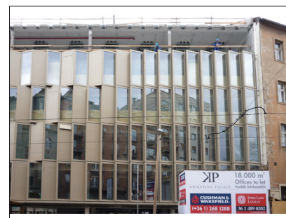
Front view of the construction site - 2009
