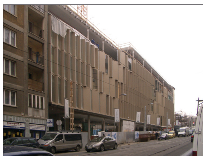
East view of the construction site - 2009
