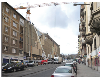
East view of the construction site - 2009
