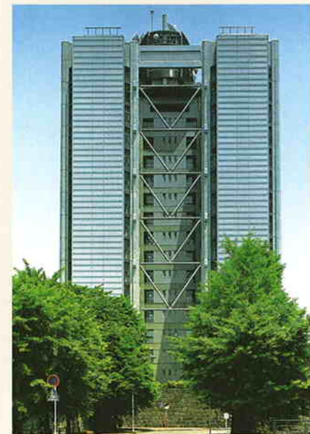
Improved earthquake resistance provided by the combination of two types of energy dissipation members Nikken Tokyo Building
