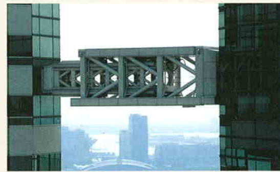
Shear panels made of low yield point steel Nissei Shin-Osaka Building
