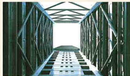
Energy dissipation members used as part of building design IK Building
