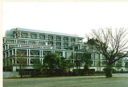
Energy dissipation members used as part of building design IK Building
