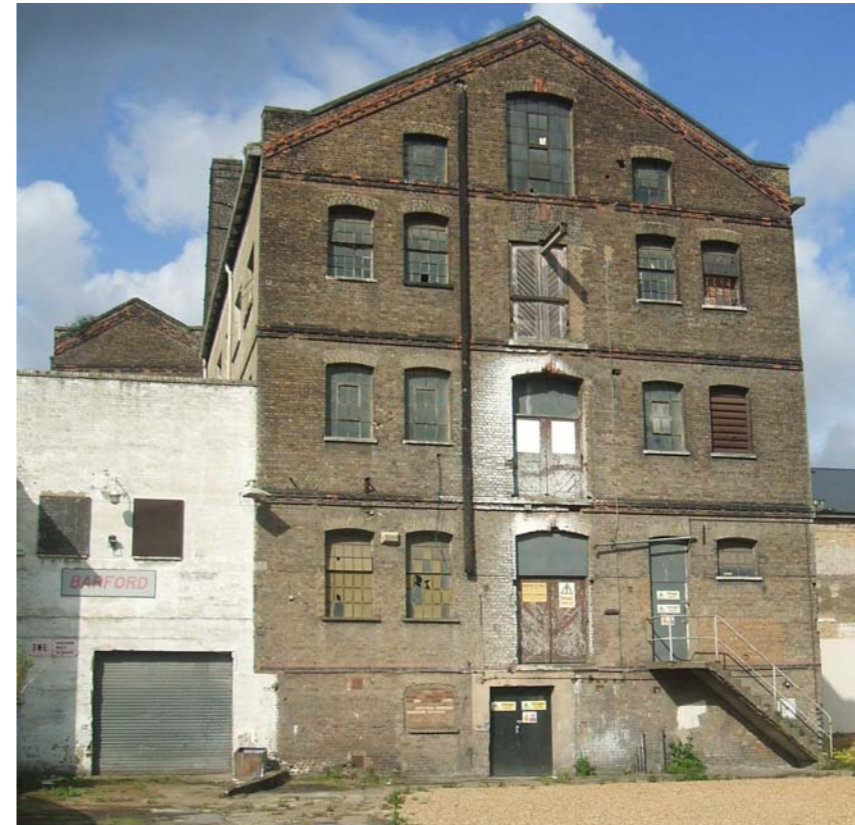
BEFORE WORK COMMENCED
