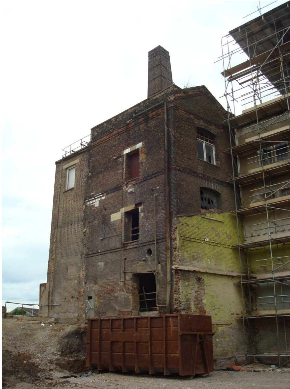
ENGINE TOWER REVEALED DURING DEMOLITION WORK
