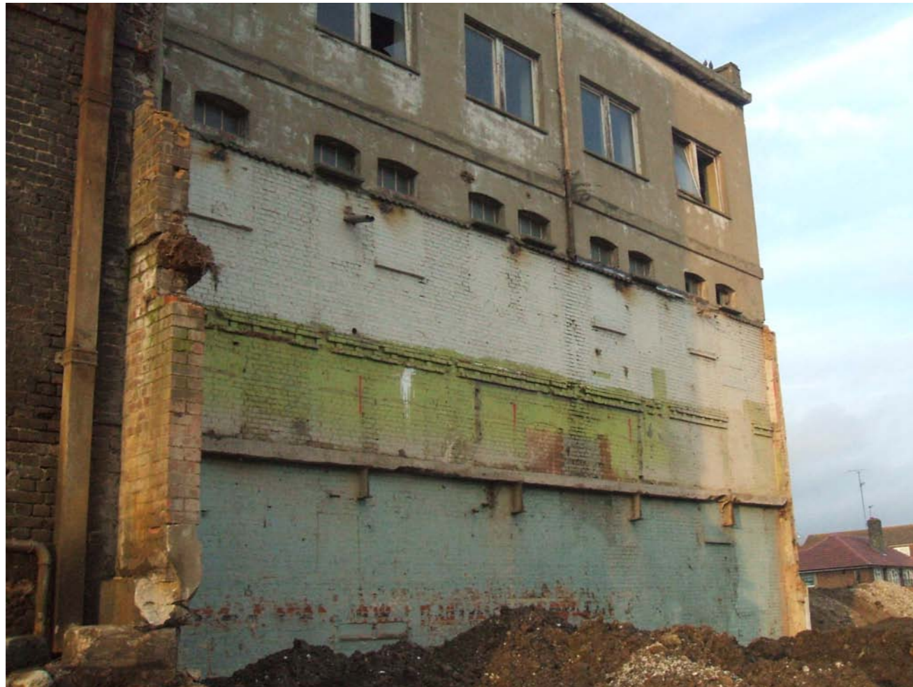
NEW COURTYARD SPACE DURING DEMOLITION OF LATER EXTENSIONS
