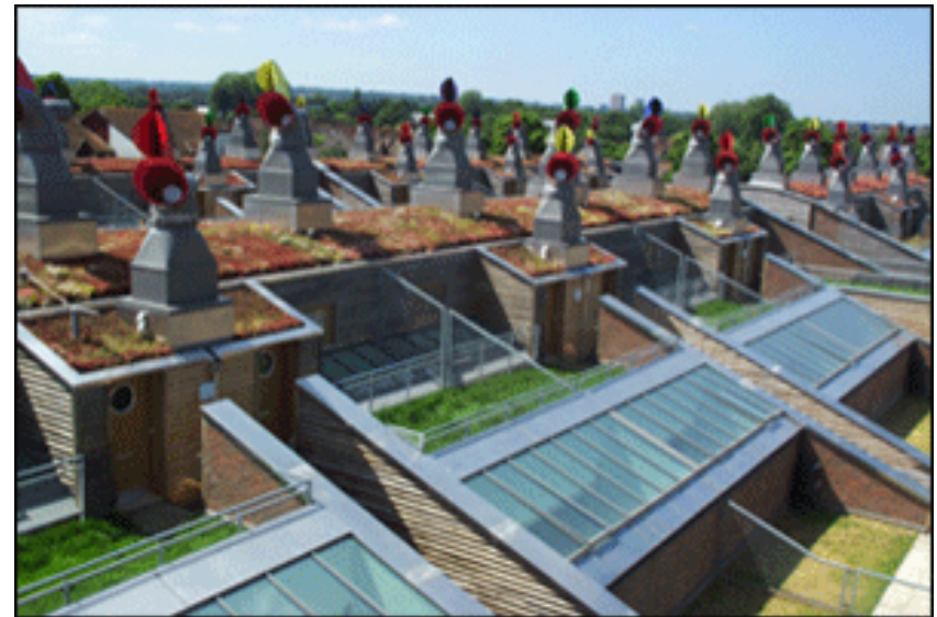
Windcatcher, BedZed Beddington Zero Energy project
