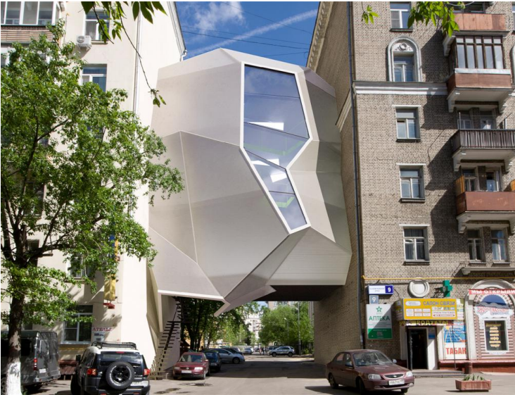
Radionica Arhitekture: Segrt Hlapic Kindergarten (CROATIA 2008)
