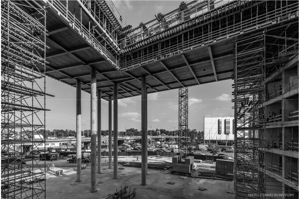
The arcade bridge structure during construction
