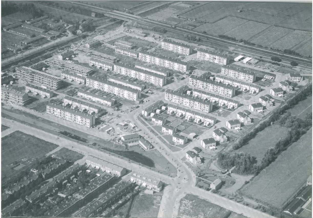
Bomenwijk under construction (early 50's), Delft Photographer unknown
