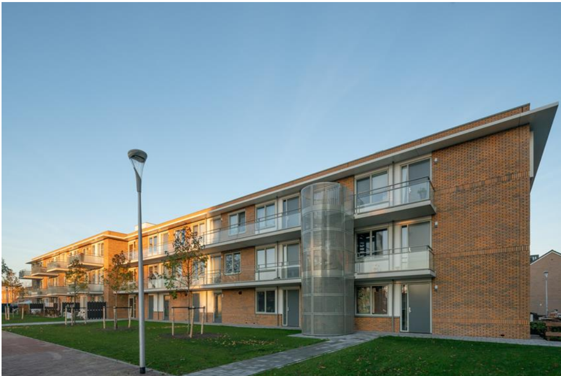
Three storey apartments, street view with bayonet and short galleries Photo by Jannes Linders
