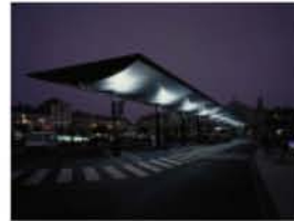
84. Bus Terminal Tours, France 1990–1992
