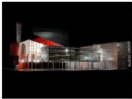
161. Treatment Plant Bergamo, Italy 2000*
