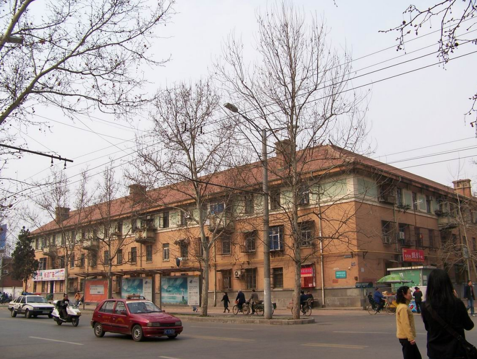
1950's worker's residential block
