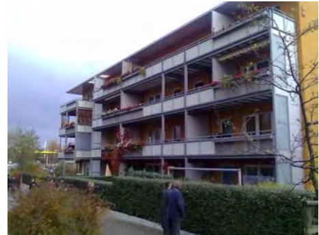
Figure 18: Dresden, housing estate rehabilitation, reducing from 6 to 3 storeys, independent terraces
