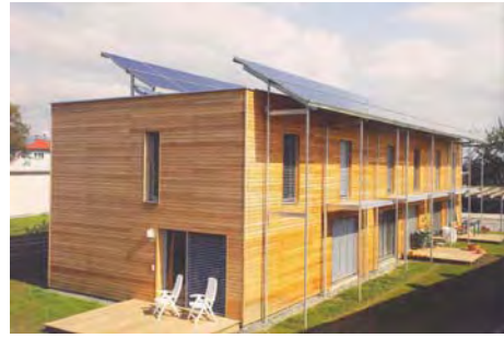
Figure 19: Passive house, Weiz, Austria
