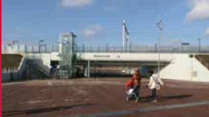
Almere Poort Station
